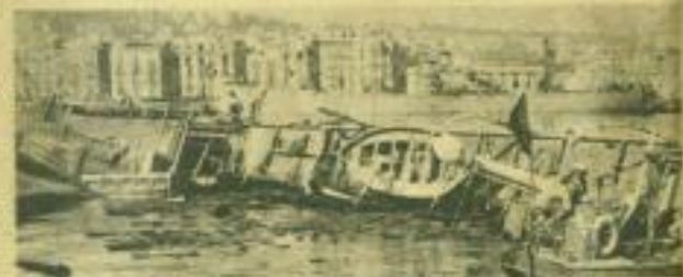
Naples harbor was heavily damaged.
