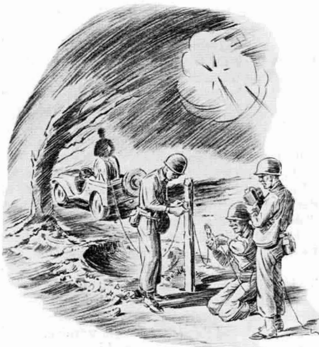
Wire crews worked day and night keeping the lines in
