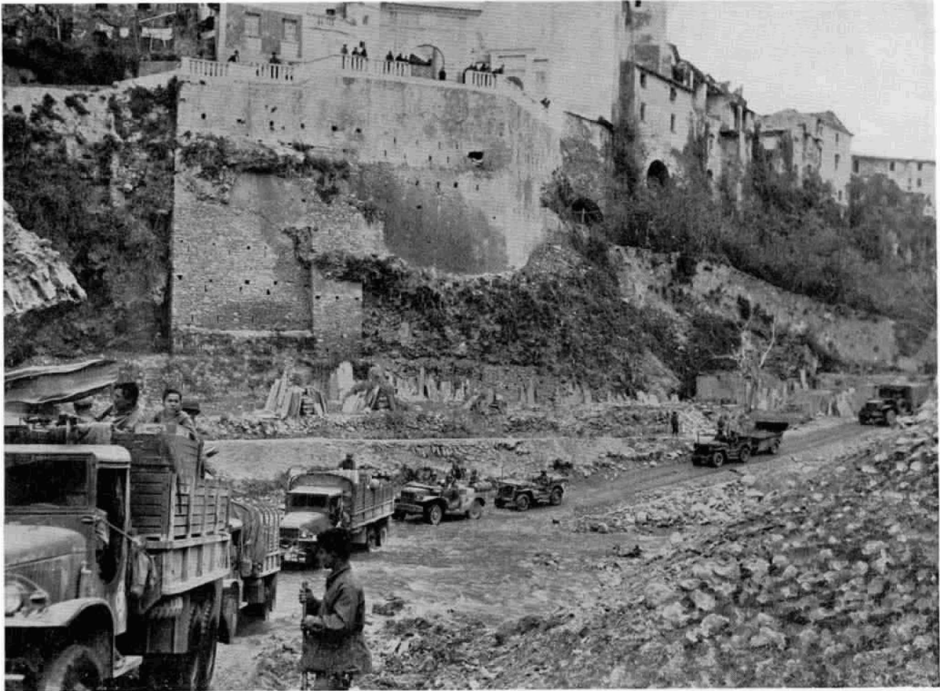
Combat Team supply convoy moves across the Frigido River over a by-pass built by the 232d Engineers
